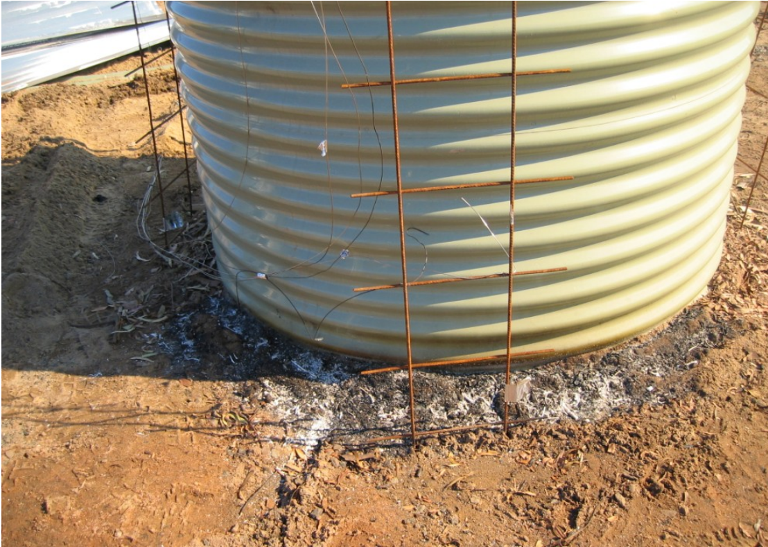
Figure C12 Tank three burnt leaf litter, no damaged to tank.
