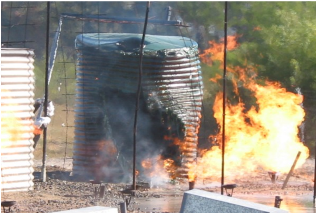
Figure C32 Tank four complete wall failure due to structural exposure.
