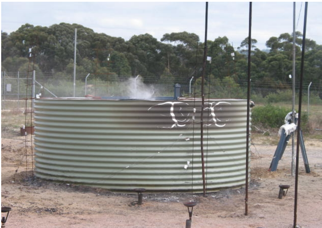
Figure C2 Tank one slight surface damage due to pre radiation.
