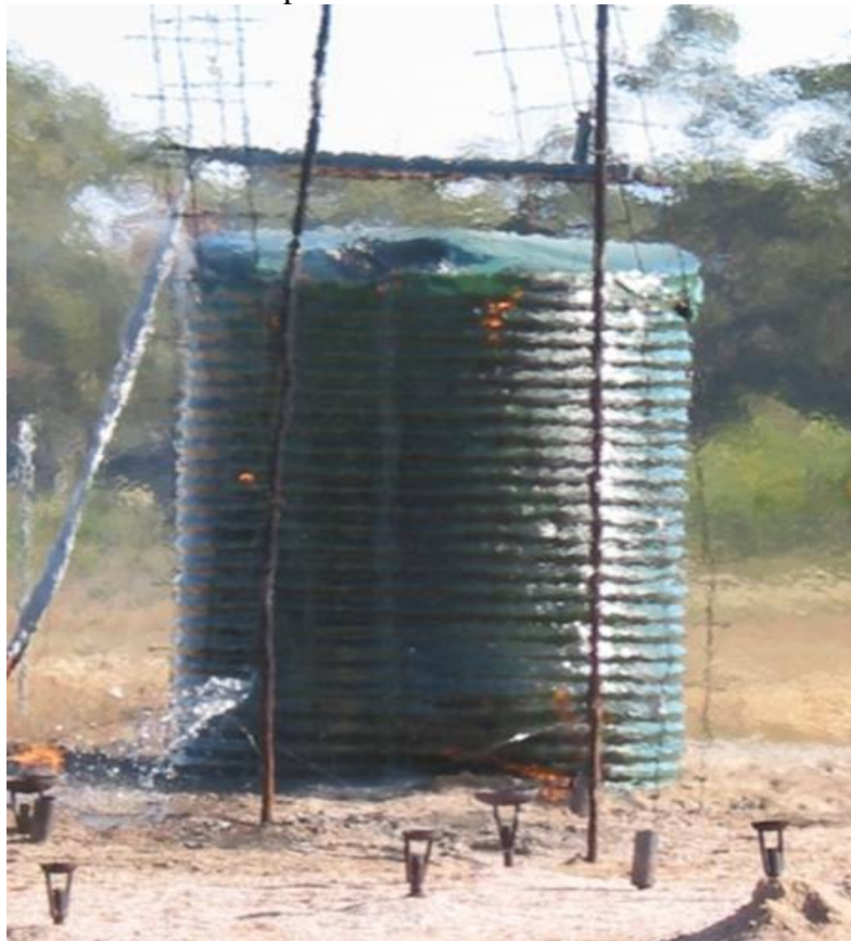
Figure C28 Tank four severely leaking due to flame exposure.
