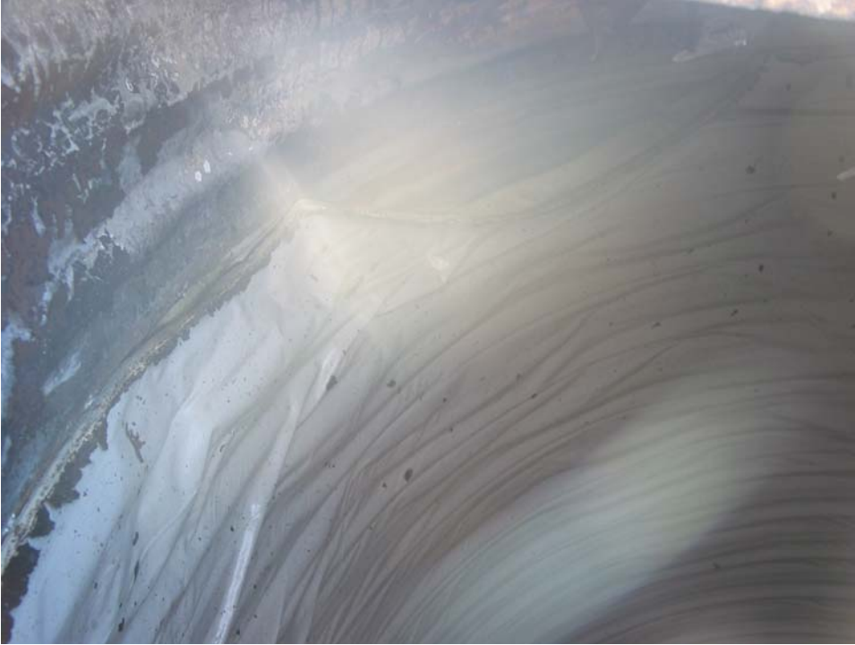
Figure 26 Liner inside tank 7
