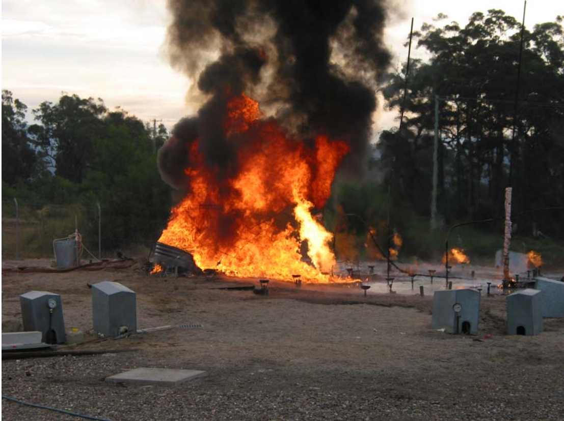
Figure C54 Tank 8 failure due to structural fire exposure.
