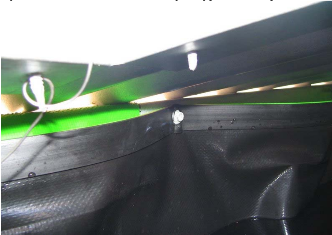
Figure C59 Bladder tank liner slightly damaged due to pre-radiation exposure.
