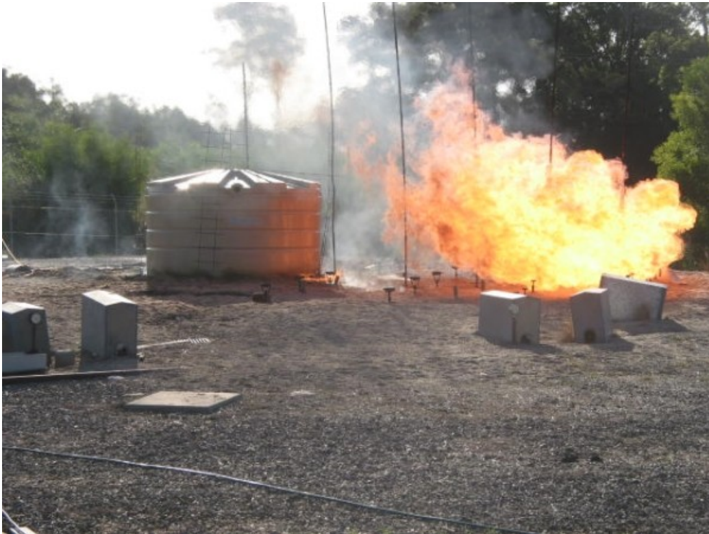
Figure C9 Tank six pre radiation exposure. Approx 25\text{Kw/m}^2
